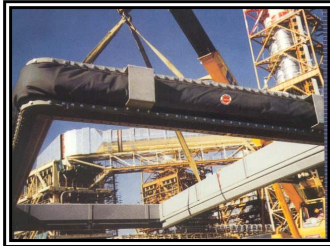
J-Flex supply a wide range of flexible products, custom made to specific requirements allowing for thermal movement; isolation of vibration and compensation for misalignment in ductwork and piping.
